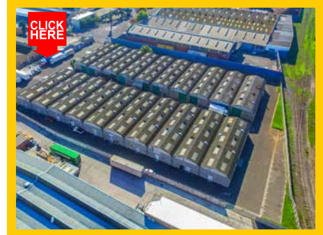
MALLEON INDUSTRIAL PARK 21 Christian Ave, Freehold
